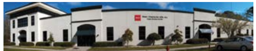
FUJIFILM Wako Chemicals U.S.A. Corp. - Cape Charles Bleeding Facility: Cape Charles,
